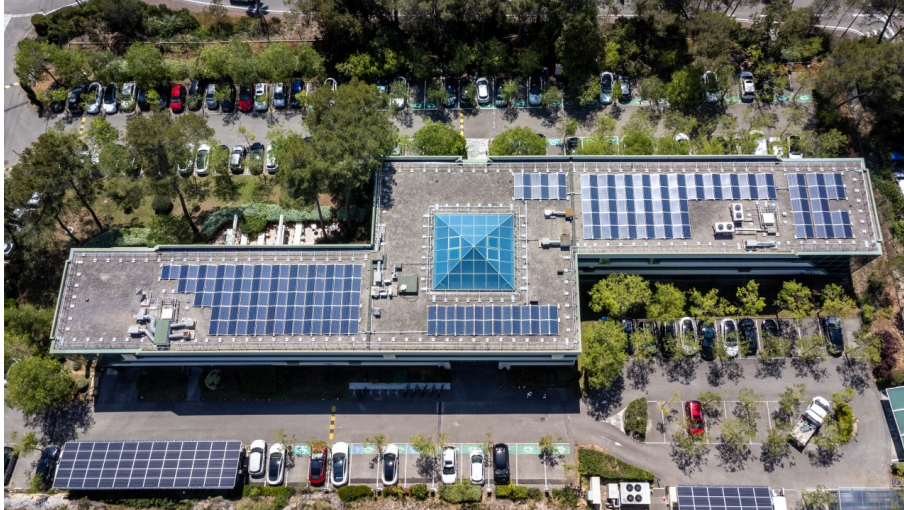
Figure 3.2: PV panel assets on the roof and in the parking area of SAP Labs, located in Mougins, France. Currently, the energy produced by PV panels is used as the building’s primary energy source.
